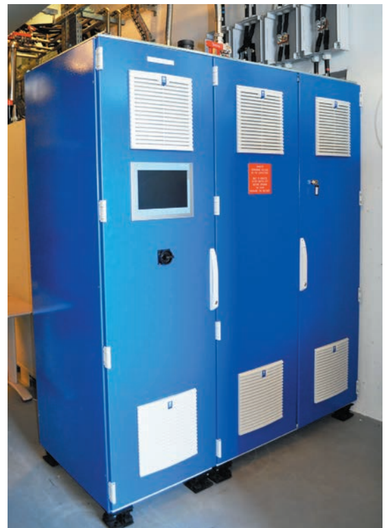
Fig. 165: The H-bridge of the new RIPS for the booster.
