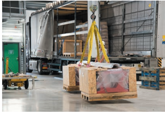
Fig. 2: The first EBS girder was delivered to the Chartreuse Hall in October 2016.
