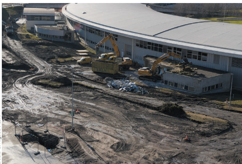
Fig. 1: Demolition of sector buildings.
